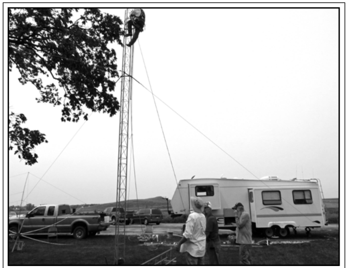
Assembling the radio tower Photo by Ed Gray
